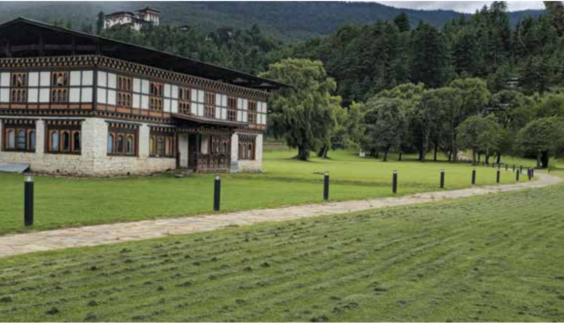
WANG PALACE, BUMTHANG, BHUTAN
